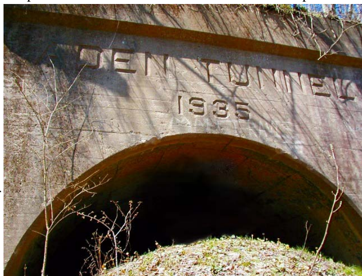
(Aden Tunnel, Carter County, 2005, ACE.) (Continued on page 3)
