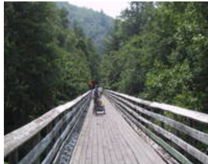
(One of the 38 bridges on the Virginia Creeper, 2005, K. Lovan)
